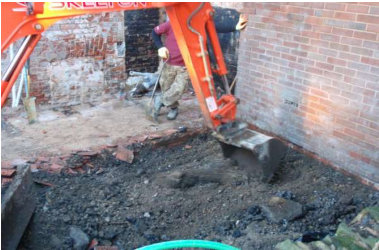
Plate 5. The site showing site reduction
