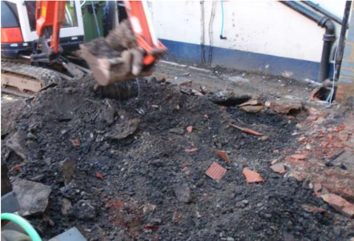
Plate 4. The site showing removing of overburden
